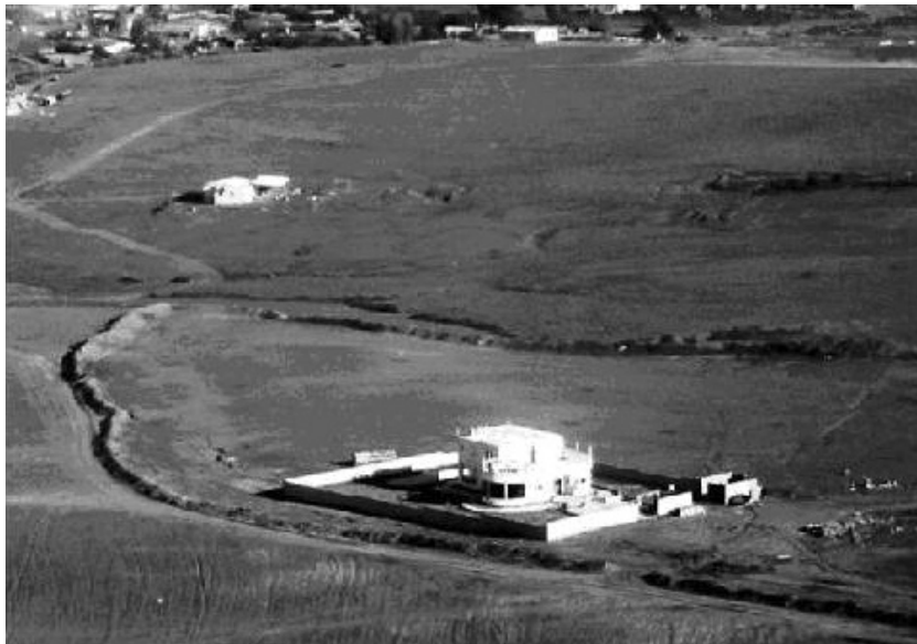
Illegal estate on state lands. Courtesy of the Ministry of Interior— National Unit for Planning, Law Supervision and Enforcement.
