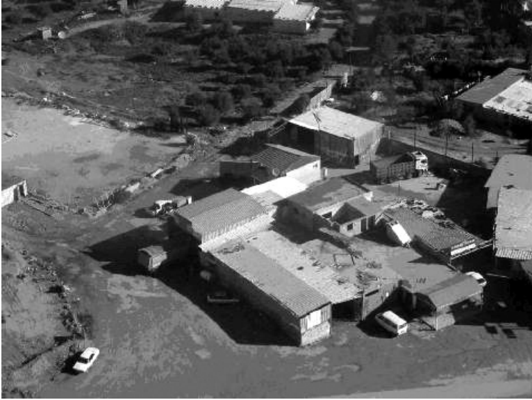
Illegal commercial constructions. Courtesy of the Ministry of Interior— National Unit for Planning Law Supervision and Enforcement.
